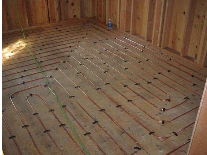
Figure 1 ARH Piping Layout
